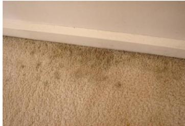
Tell-tale signs of a broken pipe or leaking water to a wall adjacent or inside/behind the wall.
